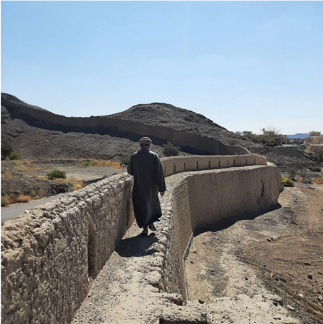
View of a restored section of the Bahla town-wall in early 2023. Photo: Maria Popp.
